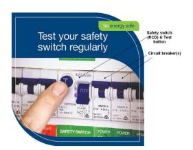
**To test your safety switch (RCD):** Press the Test or "T" button. This should automatically trip the switch to the 'OFF' position.
